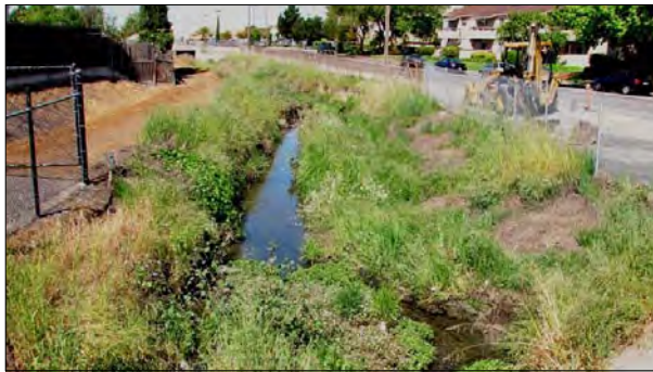
Before: Eroded channel banks along Line C near East 14th and 159th Avenue, San Leandro (Zone 2).
