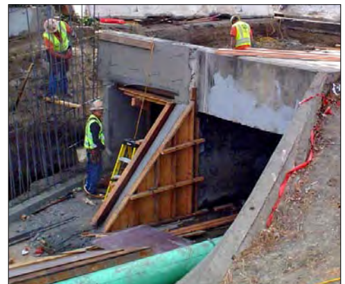
A box culvert was added on to the existing box culvert along Line F-1 at the Sycamore Street crossing, Newark (Zone 5).
