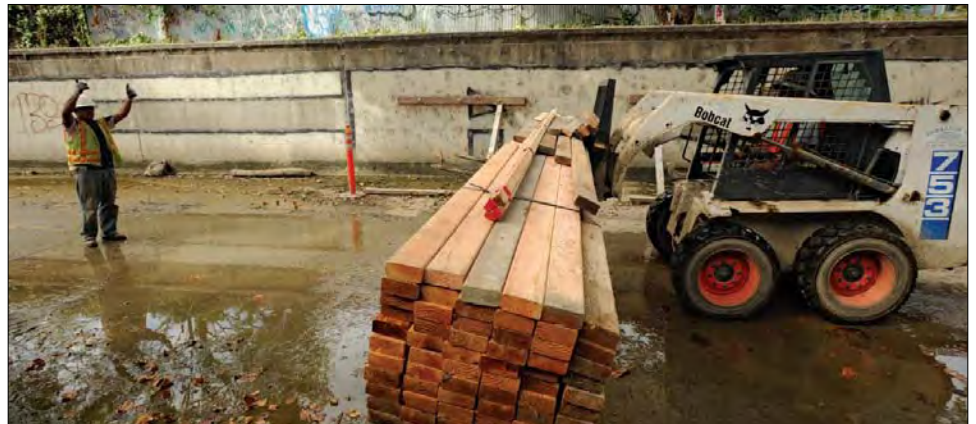
Water from the San Leandro Creek (Line P) flood channel was re-routed to another channel upstream during floodwall construction, Oakland (Zone 12).
