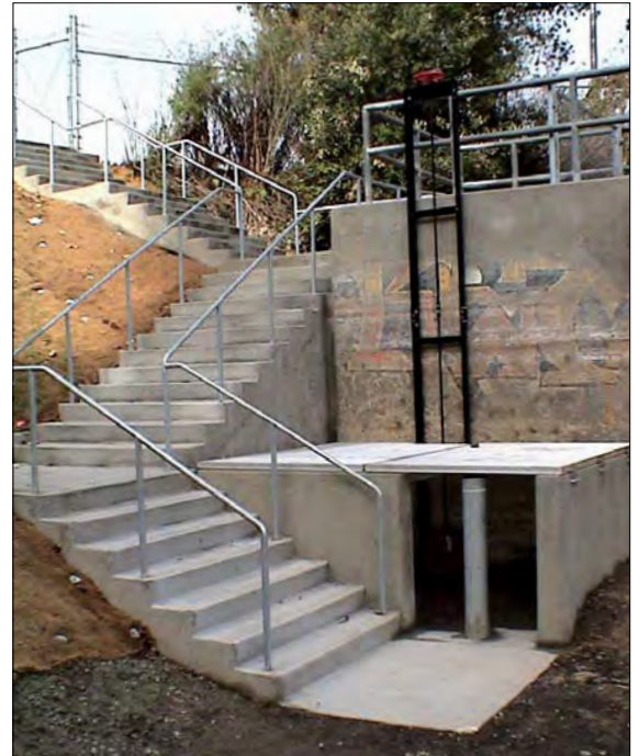
After: The new stairway and housing for control mechanism that opens and closes the outlet pipe opening; a debris trap was installed to minimize clogging of the pipe inlet, Oakland (Zone 12).
