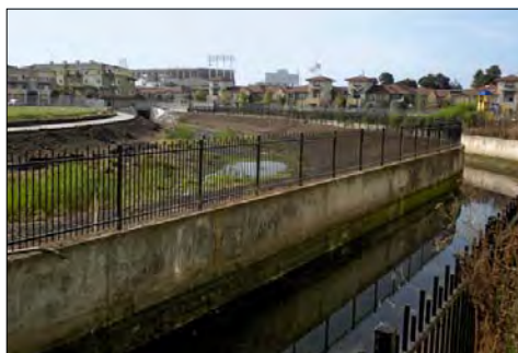
Looking downstream from Lion Way, the natural bypass creek (left) follows the curve of the Line J flood channel (right), Oakland (Zone 12).
