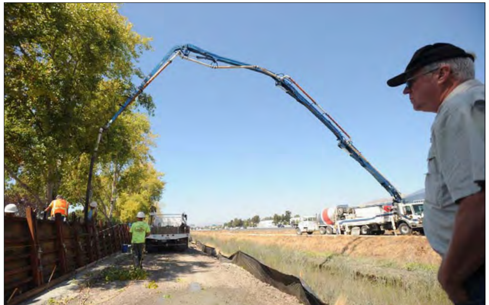
In summer, only a small amount of water flows through the Line C channel, making it an ideal time to construct a new floodwall, and stabilize and heighten the levee along the channel banks, Fremont (Zone 6).
