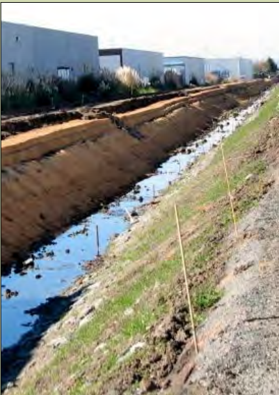
Line A channel restoration to repair eroded bank, Hayward (Zone 4).
