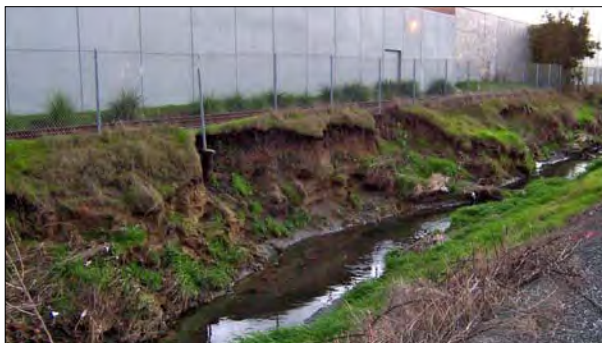
Before: Line A eroded channel banks between Cabot Boulevard and the Union Pacific Railroad, Hayward (Zone 4).
