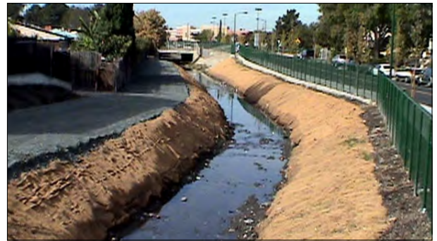
After: Line C channel banks were repaired to increase stormwater capacity, San Leandro (Zone 2).
