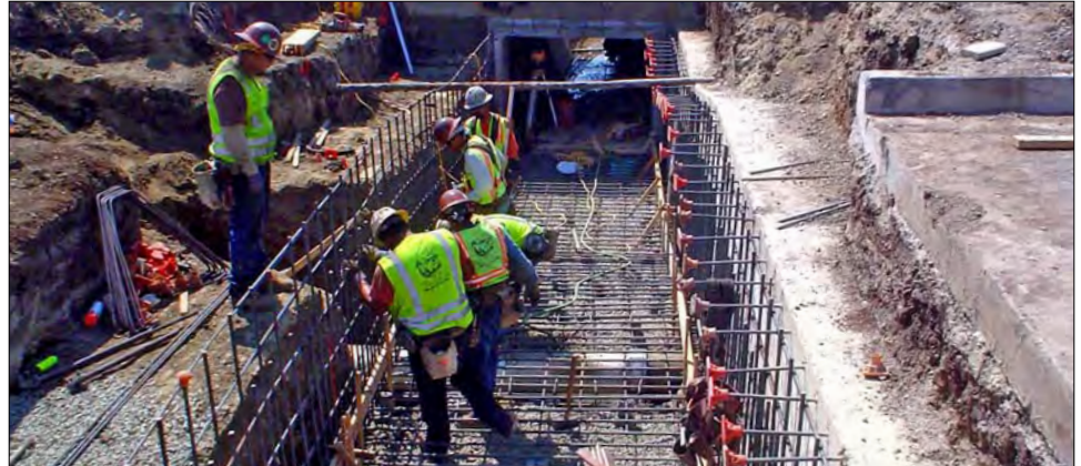
A new box culvert was added parallel to the existing box culvert along Line F-1 at the Cherry Street crossing, Newark (Zone 5).
