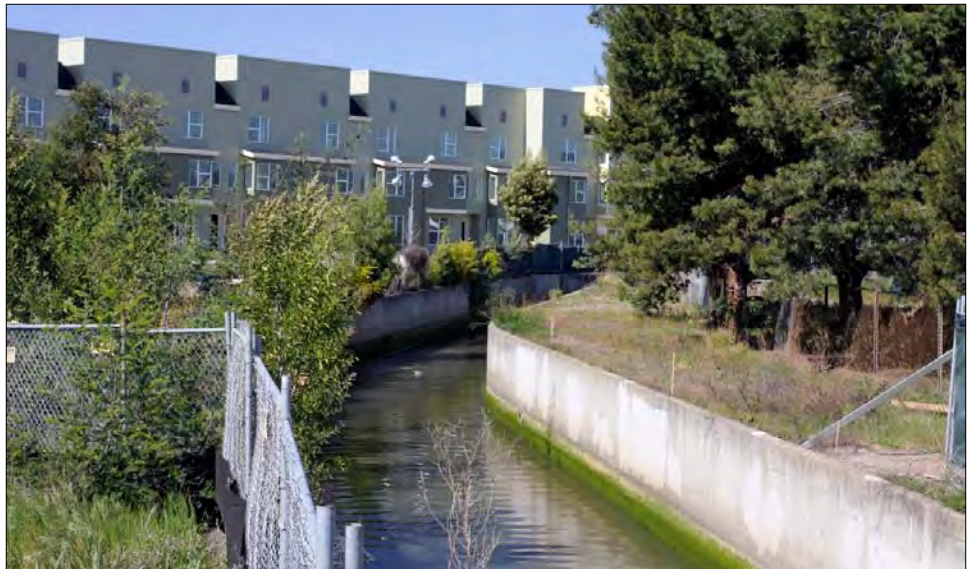
A new, natural bypass creek, which runs parallel to the Line J concrete-lined flood channel, has been created near the Lion Creek Crossing Residential Development, Oakland (Zone 12).
