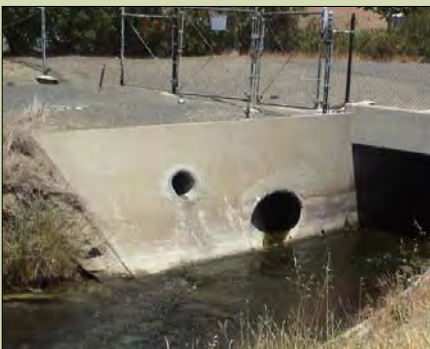
To reduce maintenance, a box culvert was removed on an abandoned section of Filbert Street along Line F-1, Newark (Zone 5).
