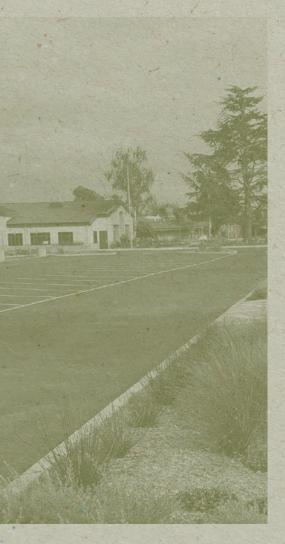
Low-impact development (LID) features slow down and redirect water into the ground or to retention areas where it can be absorbed by plants, trees, or special bioretention soil. Stormwater stays within the confines of the site, rather than running off into drains that feed into nearby waterways.
